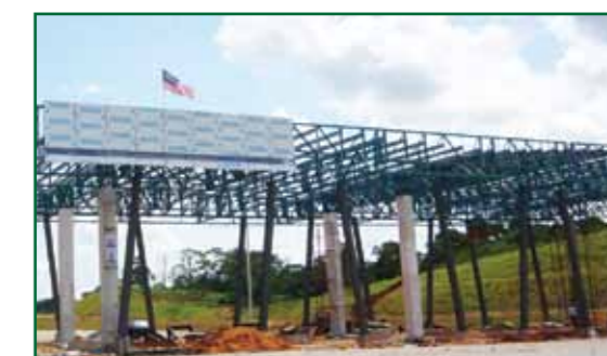
Structural Steel Frame For Toll Plaza
