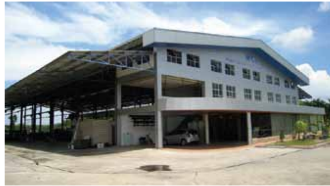
MCI office & factory
